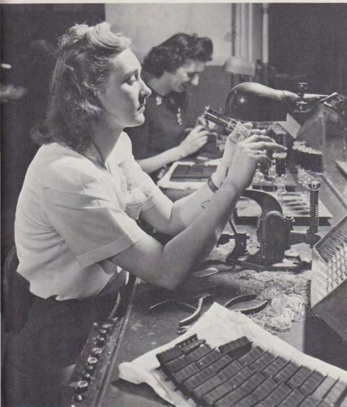
That's a vacuum tube she's working on, which should help you narrow down the time frame. We have no precise year for the photo, but we do know it was taken sometime during WWII at one of Western's two tube shops.
