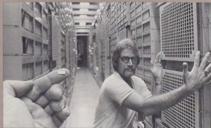
In this shot posed in a Long Lines office at the end of the decade, the pace of technological change is dramatically displayed. The tiny chip, from a 3B Processor, contains the equivalent memory of the large units indicated by the man's outstretched hands.
