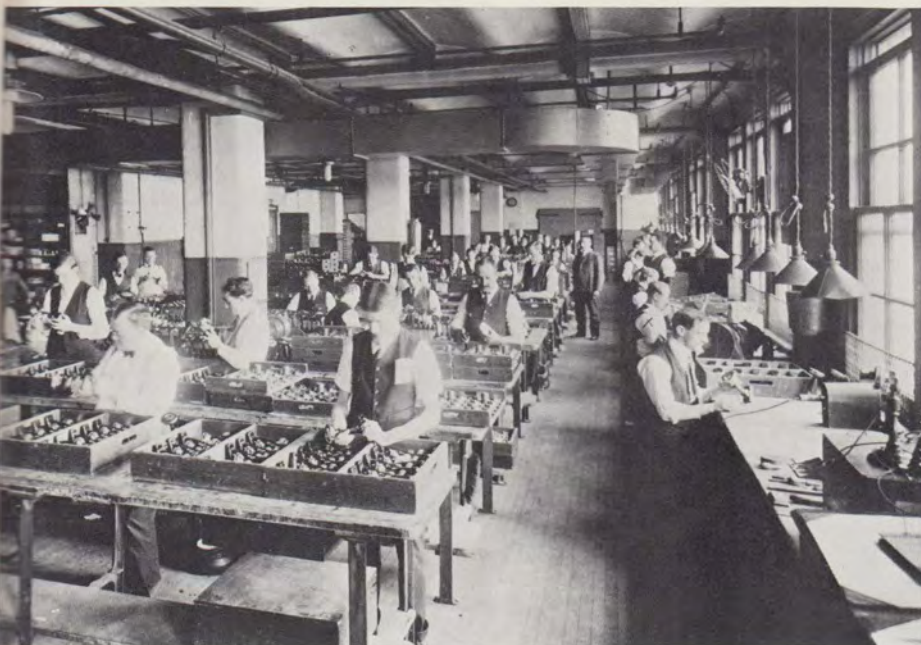
1905 —The term “mass production” hadn’t taken on meaning yet. These workers are assembling telephone transmitters. The workers in the 1895 photo (left) would have experienced no future shock in this shop.
