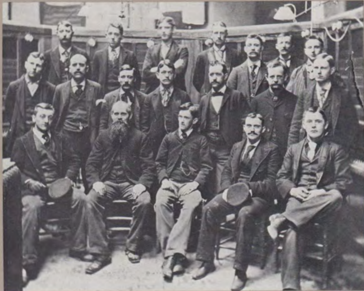
Group photos were taken for every event it seems. This is the installation crew that replaced the switchboard at Louisville after a fire in 1897.
